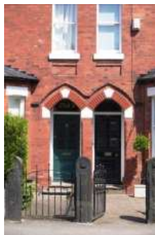
Original doors along Oldfield Road at nos. 48-58
