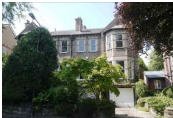
Example of the houses along Burlington Road, showing the leafy character of the street but also the inappropriate introduction of basement garages.
