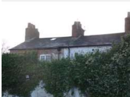
The rear elevations of cottages at 1-11 Sandiway Road beyond a substantial brick wall. Note that some cottages have been painted.
