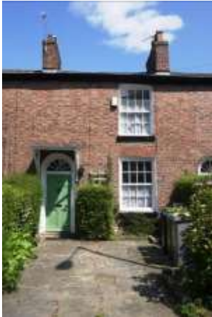
Example of the cottages on Sandiway Road. Note the inappropriate asphalt-covered porch and the loss of the front garden.
