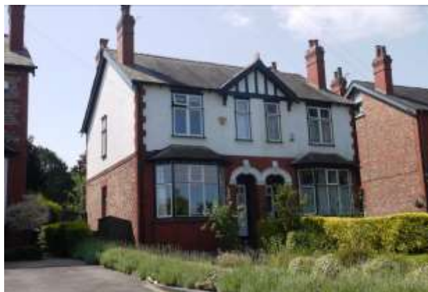
The palette of materials used across the Conservation Area include slate roofs and red brick, half-timbering, stained glass and leaded-lights, timber windows, clay chimney pots. Pebble-dash can be found along Oldfield Road but is not common.
