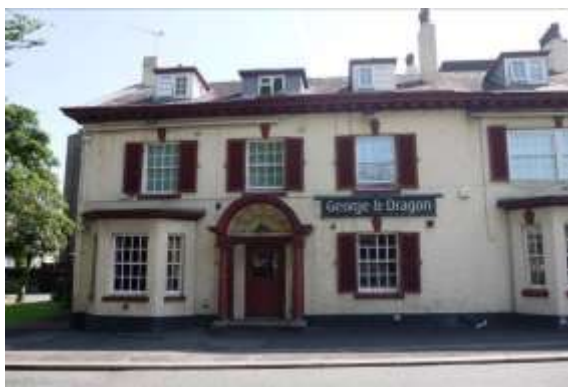
The original elevation of the George and Dragon, late 18 th century in date
