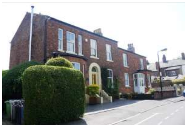
Edale House and Rose Lea showing good quality buildings with some inappropriate alterations and loss of boundary walls.
