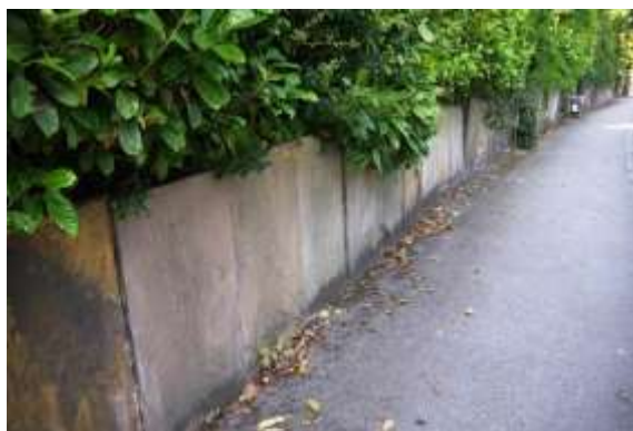
Boundary treatment of upturned slabs along Oldfield Road
