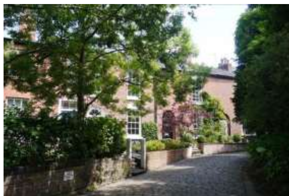
Cottages within a green setting with replacement stone setts
