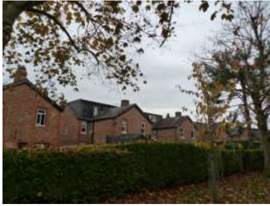
The rear of properties on the north side of Oldfield Road
