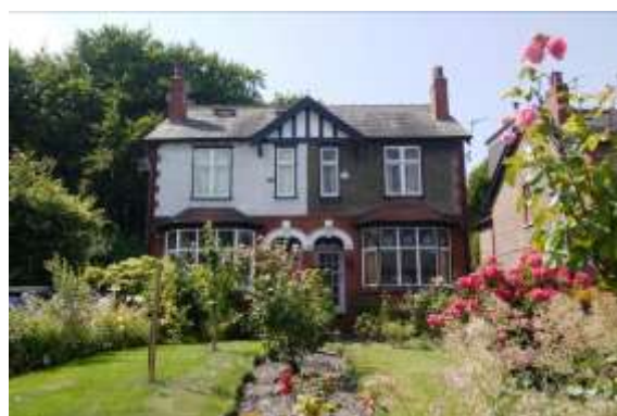
Original windows with leaded glazing and stained glass at nos. 1-3
